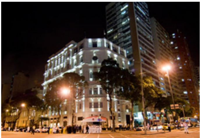
Navy Club building located in Downtown of Rio de Janeiro
